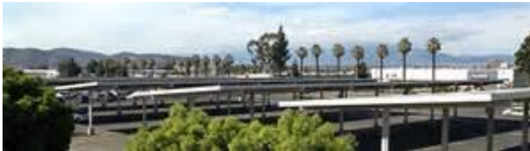
Figure 15. Solar Cells Functioned as Parking Roof at the University of California, Riverside, USA, SIGI Project (Courtesy of UC Riverside)
